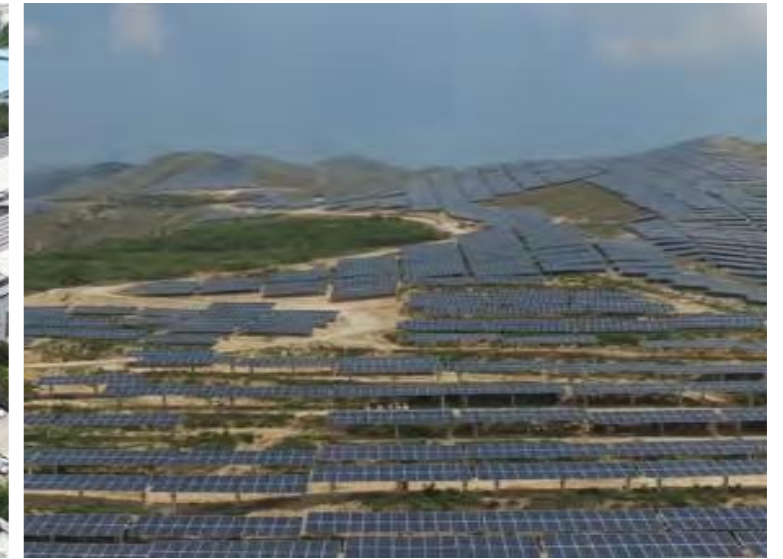
20WM Solar System In France
